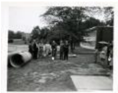
Leo Urbanske at a Groundbreaking (214-02-01-9233)
