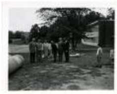
Leo Urbanske at a Groundbreaking (214-02-01-9237)
