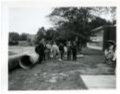
Leo Urbanske at a Groundbreaking (214-02-01-9228)
