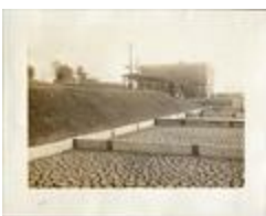
"Laboratory Disposal Plant" (21-01-01-13-5154)
