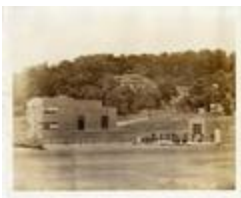
Water Pollution Control Plant (21-01-01-13-5153)
