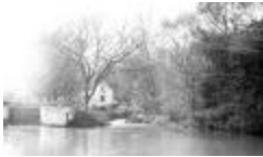
C&O Canal Lock and Lockhouse (123-02-03-0152)
