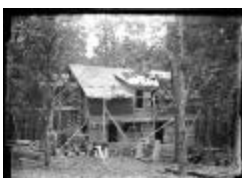
The Jewett Home Under Construction (123-02-06-0077)
