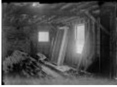
Interior of the Jewett Home Under Construction (123-02-06-0078)
