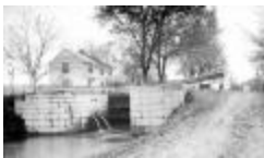
C&O Canal Lock and Lockhouse (123-02-03-0155)
