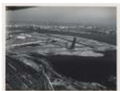
Washington National Airport (13-06-03-5092)
