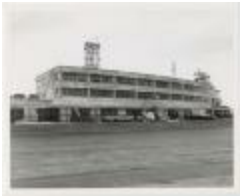
Portion of Terminal A (13-06-03-5094)
