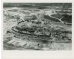
Construction of Washington National Airport's Terminal A (13-06-03-5087)
