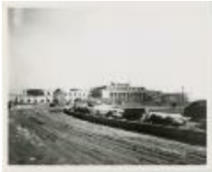
Building Terminal A (13-06-03-5077)
