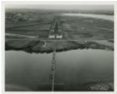
Washington National Airport Runway (13-06-03-5073)
