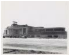
Construction of Terminal A (13-06-03-5099)
