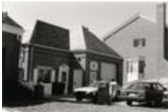
Arlington County Fire Station 7 Fairlington, 1996 (202-6146)
