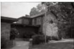
Dawson-Bailey House, rear addition, 1997 (250-01-01-1181)
