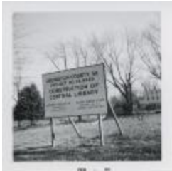
Arlington Central Library Construction (29-01-13-01-0058)
