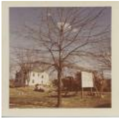
Central Library Construction Site (29-01-13-01-0062)
