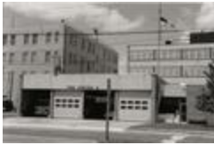
Arlington County Fire Station 4 Clarendon, 1996 (202-6143)
