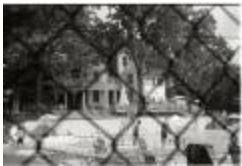
Febrey-Kincheloe House, through pool fence, 1997 (250-01-01-1307)
