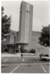
St. Charles Borromeo Catholic Church, 1996 (202-6101)
