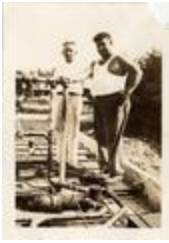
Inspection of Water Treatment Plant (21-01-01-15-5166)
