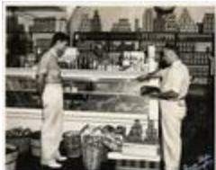
Grocery Store Inspection (21-01-01-15-5163)
