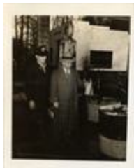
Inspection of Oil Tank, 1943 (21-5323)
