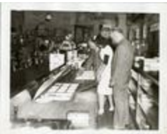
Inspection of Soda Fountain (21-5240)
