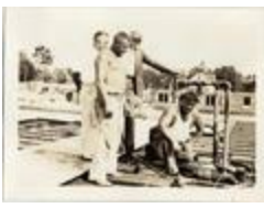
Inspection of Water Treatment Plant (21-01-01-15-5165)
