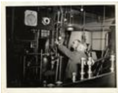
Inspection of Equipment in Pasteurizing Plant, 1943 (21-5300)
