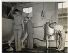
Inspection of Pasteurizing Plant (21-01-01-13-5157)
