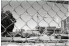
Construction on Wilson (250-09-01-8788)
