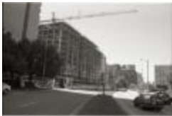
Construction on Fairfax Drive (250-09-01-8791)
