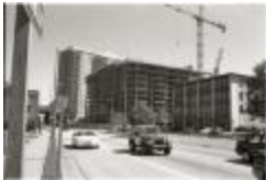
Construction on Fairfax Drive (250-09-01-8792)
