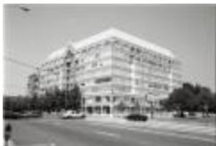
Quincy Street Station (250-06-01-3606)
