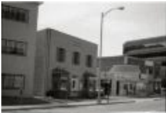
The Loflin Building (250-03-01-2890)
