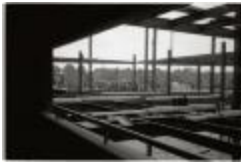
Hecht Company Office Tower Construction (250-05-01-3547)
