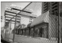
Closed Strip Mall on Courthouse Road (250-03-01-2877)
