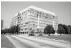
Quincy Street Station (250-06-01-3607)
