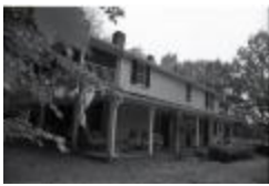
Basil Hall House Front Porch (250-08-01-8747)
