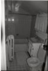
Basil Hall House Bathroom (250-08-01-8761)
