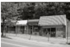
Closed Strip Mall on Courthouse Road (250-03-01-2879)
