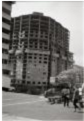
Construction of Arlington Courthouse Place (250-03-01-2883)
