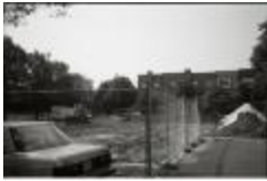
Construction on Quincy Street (250-05-01-3555)
