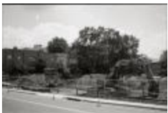
Demolition of 1110 and 116 Quincy Street (250-05-01-3543)
