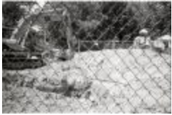
Fixing Water Main at Woodmont (250-05-01-3540)
