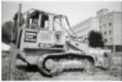
Dominion Front Loader on Site (250-05-01-3558)
