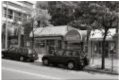
Closed Strip Mall on Courthouse Road (250-03-01-2880)
