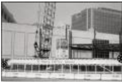
Hecht Company Office Tower Construction (250-05-01-3550)
