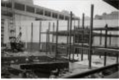
Hecht Company Office Tower Construction (250-05-01-3548)
