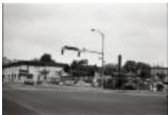
Construction of Eckerd Pharmacy (250-09-01-8772)
