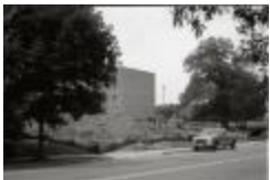
Demolition of 1110 and 116 Quincy Street (250-05-01-3542)
