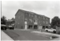
Construction of Arlington Heights Townes (250-09-01-8773)
