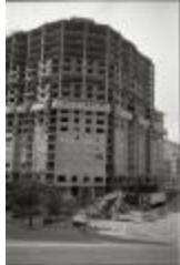
Construction of Arlington Courthouse Place (250-03-01-2884)
