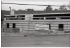
Construction of Barcroft Sports & Fitness Center (250-09-01-8769)
