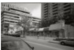
Closed Strip Mall on Courthouse Road (250-03-01-2878)
