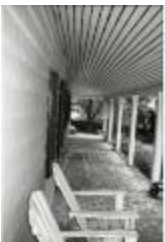
Basil Hall House Front Porch (250-08-01-8766)
