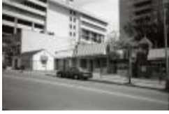
Closed Strip Mall on Courthouse Road (250-03-01-2881)
