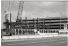
Hecht Company Office Tower Construction (250-05-01-3551)
