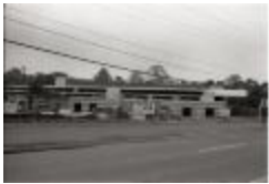
Construction of Barcroft Sports & Fitness Center (250-09-01-8770)
