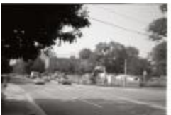
Construction on Quincy Street (250-05-01-3554)
