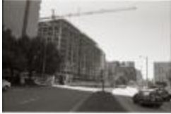
Construction on Fairfax Drive (250-09-01-8791)
