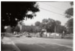
Construction on Quincy Street (250-05-01-3554)
