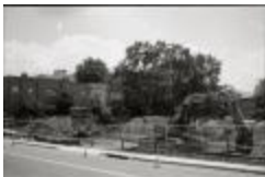
Demolition of 1110 and 116 Quincy Street (250-05-01-3543)
