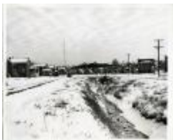
Open Drain in Snow (32-07-07-17-0133)
