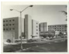
Hospital From Street, Two Light Poles (32-04-11-12-0121)
