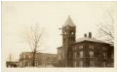
Arlington County Courthouse (100-03-01-0401)
