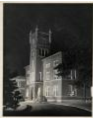
County Courthouse at Night (100-03-01-0420)
