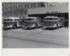
Fire Engines at Station No. 4 (100-01-03-0363)
