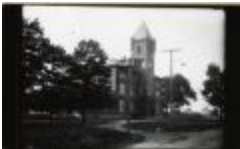
Arlington County Courthouse (100-03-01-0403)
