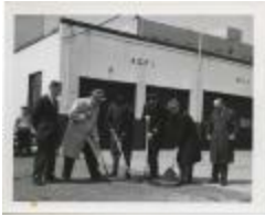
Fire Station #4 Groundbreaking (100-01-03-0238)
