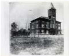
Arlington County Courthouse (100-03-01-0402)
