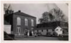
Arlington County Courthouse (100-03-01-0408)
