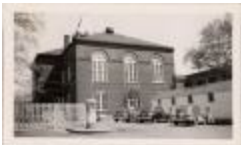
Arlington County Courthouse (100-03-01-0416)
