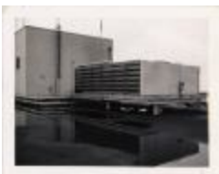
Air Conditioning Tower on the Courthouse Roof (100-03-01-0406)
