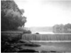
Washington Aqueduct Dam (123-02-14-0116)
