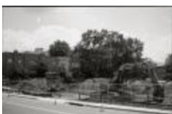
Demolition of 1110 and 116 Quincy Street (250-05-01-3543)
