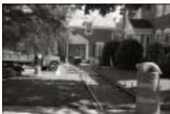
New Sidewalks at Fairlington Commons (250-09-01-8781)
