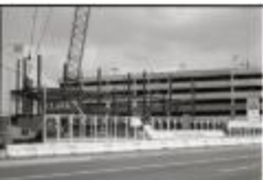
Hecht Company Office Tower Construction (250-05-01-3551)
