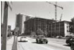
Construction on Fairfax Drive (250-09-01-8792)
