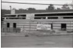
Construction of Barcroft Sports & Fitness Center (250-09-01-8769)
