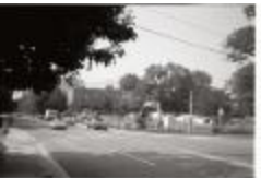
Construction on Quincy Street (250-05-01-3554)
