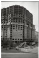
Construction of Arlington Courthouse Place (250-03-01-2884)
