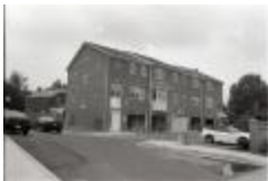
Construction of Arlington Heights Townes (250-09-01-8773)
