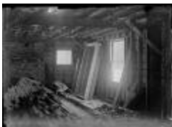
Interior of the Jewett Home Under Construction (123-02-06-0078)
