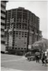
Construction of Arlington Courthouse Place (250-03-01-2883)
