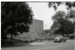
Demolition of 1110 and 116 Quincy Street (250-05-01-3542)
