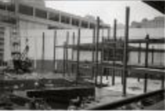
Hecht Company Office Tower Construction (250-05-01-3548)
