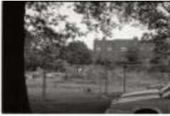
Demolition of 1110 and 116 Quincy Street (250-05-01-3544)
