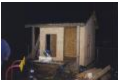
Construction at Night (332-05-08-0133)
