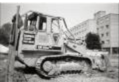
Dominion Front Loader on Site (250-05-01-3558)
