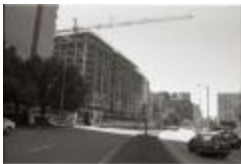
Construction on Fairfax Drive (250-09-01-8791)
