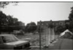
Construction on Quincy Street (250-05-01-3555)
