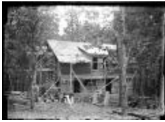
The Jewett Home Under Construction (123-02-06-0077)
