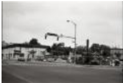
Construction of Eckerd Pharmacy (250-09-01-8772)
