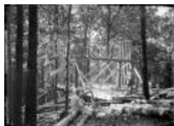
Frame of the Jewett Home Under Construction (123-02-06-0070)
