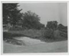
Future site of the Arlington County Central Library (29-01-13-01-0060)
