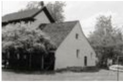
Ball-Sellers House, Original Structure, 1996 (202-6240)
