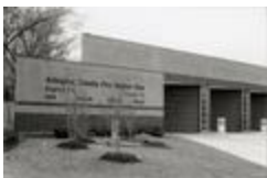
Arlington County Fire Station 1 Glebe Road, 1996 (202-6138)
