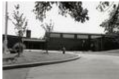
Claremont Elementary School, 1996 (202-6153)
