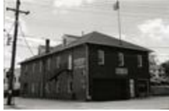
Arlington County Fire Station 3 Cherrydale, 1996 (202-6141)
