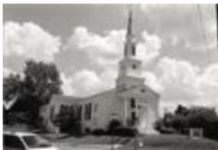
Walker Chapel United Methodist Church, 1996 (202-6121)
