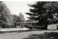
Nottingham Elementary School, 1996 (202-6171)
