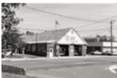
Arlington County Fire Station 6 Falls Church, 1996 (202-6145)
