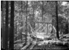
Frame of the Jewett Home Under Construction (123-02-06-0070)
