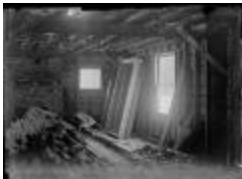
Interior of the Jewett Home Under Construction (123-02-06-0078)
