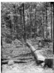
Cleared Area for the Jewett Home (123-02-06-0074)
