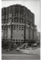
Construction of Arlington Courthouse Place (250-03-01-2884)
