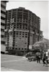
Construction of Arlington Courthouse Place (250-03-01-2883)
