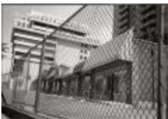
Closed Strip Mall on Courthouse Road (250-03-01-2877)
