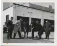
Fire Station #4 Groundbreaking (100-01-03-0238)
