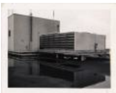
Air Conditioning Tower on the Courthouse Roof (100-03-01-0406)
