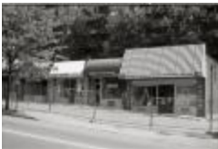
Closed Strip Mall on Courthouse Road (250-03-01-2879)
