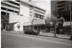
Closed Strip Mall on Courthouse Road (250-03-01-2881)
