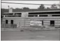
Construction of Barcroft Sports & Fitness Center (250-09-01-8769)
