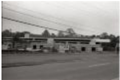
Construction of Barcroft Sports & Fitness Center (250-09-01-8770)
