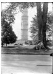
Washington Monument Under Construction (123-02-16-0048)
