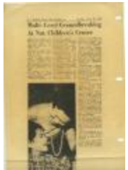
Northern Virginia Sun March 23, 1972 "Syphax Groundbreaking National Children's Center" (196-03-23-1972)
