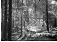
Frame of the Jewett Home Under Construction (123-02-06-0070)
