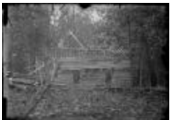
The Jewett Home Under Construction (123-02-06-0066)
