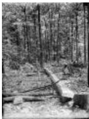
Cleared Area for the Jewett Home (123-02-06-0074)
