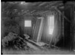
Interior of the Jewett Home Under Construction (123-02-06-0078)
