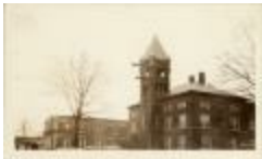
Arlington County Courthouse (100-03-01-0401)
