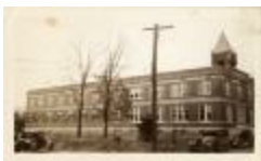
Arlington County Courthouse (100-03-01-0405)
