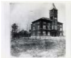
Arlington County Courthouse (100-03-01-0402)
