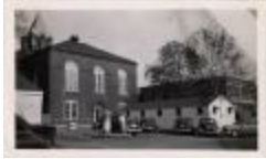
Arlington County Courthouse (100-03-01-0408)
