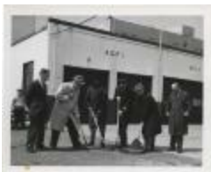
Fire Station #4 Groundbreaking (100-01-03-0238)
