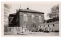
Arlington County Courthouse (100-03-01-0416)
