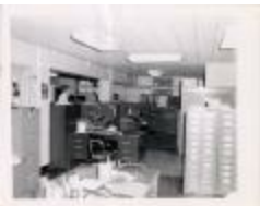
Courthouse Basement, South Wing, IBM section (100-03-01-0425)
