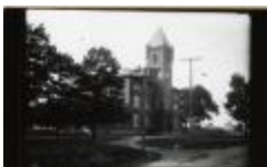
Arlington County Courthouse (100-03-01-0403)
