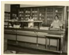
Restaurant serving line, 1940 (21-5380)
