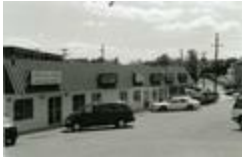
Shopping Center, Lee Highway Across from Fire House #3, 1996 (202-6227)
