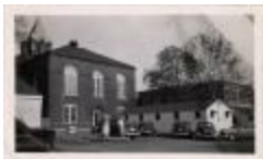
Arlington County Courthouse (100-03-01-0408)
