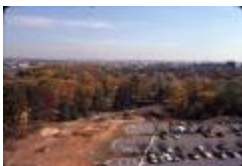
Construction Area of I-66 from Above (210-0009)
