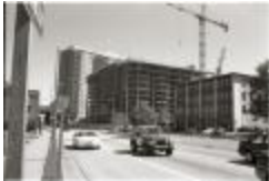
Construction on Fairfax Drive (250-09-01-8792)
