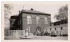
Arlington County Courthouse (100-03-01-0416)
