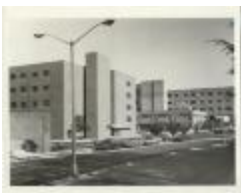
Hospital From Street, Two Light Poles (32-04-11-12-0121)
