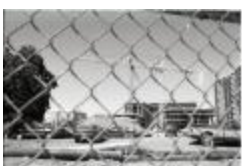
Construction on Wilson (250-09-01-8788)
