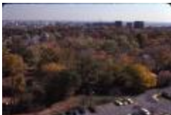
Construction Area of I-66 from Above (210-0007)
