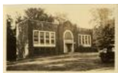
Woodmont School Building (32-07-08-01-0156)
