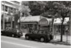
Closed Strip Mall on Courthouse Road (250-03-01-2880)
