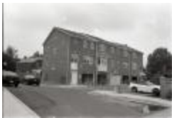
Construction of Arlington Heights Townes (250-09-01-8773)
