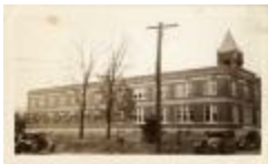
Arlington County Courthouse (100-03-01-0405)
