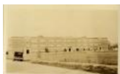
Washington-Lee School Building (32-07-08-01-0154)
