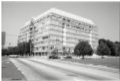
Quincy Street Station (250-06-01-3607)
