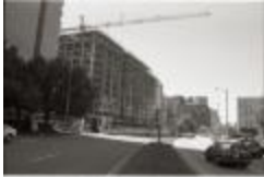
Construction on Fairfax Drive (250-09-01-8791)
