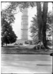
Washington Monument Under Construction (123-02-16-0048)
