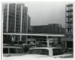
Rosslyn Pedestrian Bridge (214-03-01-9313)
