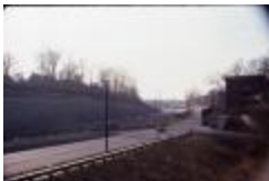
Finished I-66 West Out of Rosslyn (210-0037)
