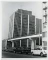
Rosslyn Pedestrian Bridge (214-03-01-9314)
