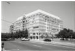
Quincy Street Station (250-06-01-3606)
