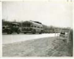
"Road Very Dangerous" (13-06-03-5110)
