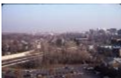
Completed I-66 from Above (210-0010)
