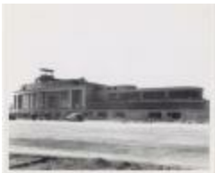
Construction of Terminal A (13-06-03-5099)
