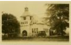
Hume School Building (32-07-08-01-0140)
