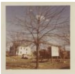
Central Library Construction Site (29-01-13-01-0062)
