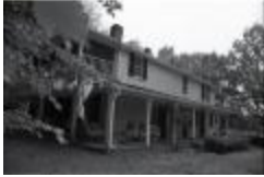
Basil Hall House Front Porch (250-08-01-8747)
