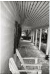
Basil Hall House Front Porch (250-08-01-8766)
