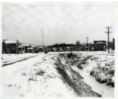
Open Drain in Snow (32-07-07-17-0133)
