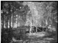
Frame of the Jewett Home Under Construction (123-02-06-0071)
