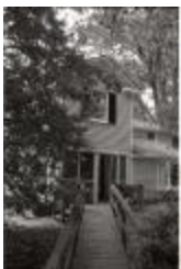
Kitchen Entrance to Basil Hall House (250-08-01-8767)
