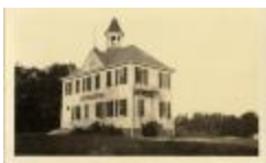
Saegmuller School Building (32-07-08-01-0151)
