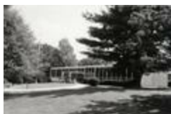
Nottingham Elementary School, 1996 (202-6171)
