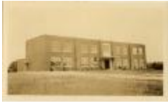
Jefferson Colored School, Main Building (32-07-08-01-0143)
