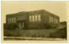
James Monroe School Building (32-07-08-01-0141)
