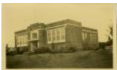
Henry Clay School Building (32-07-08-01-0139)
