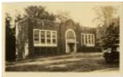
Woodmont School Building (32-07-08-01-0156)
