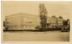
Nellie Custis School Building (32-07-08-01-0148)
