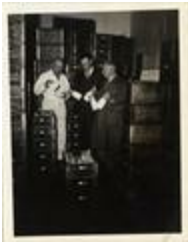
Inspection of Milk Storage Facility, 1943 (21-5304)
