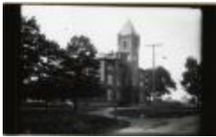
Arlington County Courthouse (100-03-01-0403)
