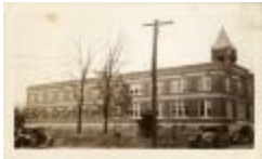
Arlington County Courthouse (100-03-01-0405)
