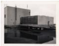
Air Conditioning Tower on the Courthouse Roof (100-03-01-0406)
