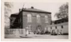
Arlington County Courthouse (100-03-01-0416)
