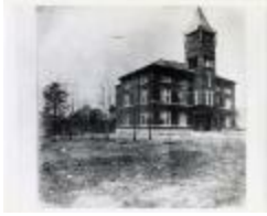
Arlington County Courthouse (100-03-01-0402)
