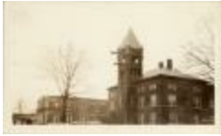
Arlington County Courthouse (100-03-01-0401)
