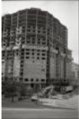
Construction of Arlington Courthouse Place (250-03-01-2884)
