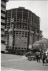
Construction of Arlington Courthouse Place (250-03-01-2883)
