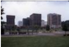
Rosslyn Circle Bus Terminal (210-0029)
