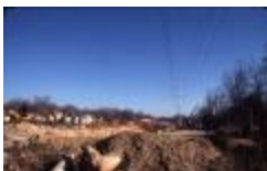
Construction of I-66 Near McKinley Road (210-0012)
