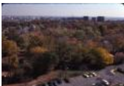
Construction Area of I-66 from Above (210-0007)
