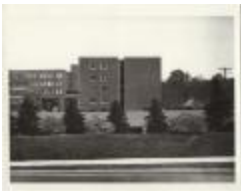
Hospital From Street, Garage (32-04-11-12-0120)
