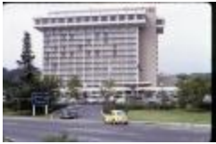
Newer Marriott Hotel at Key Bridge (210-0034)
