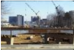
Construction of the George Mason Bridge (210-0042)
