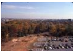
Construction Area of I-66 from Above (210-0009)
