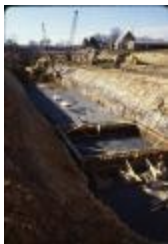
Pouring Concrete for I-66 (210-0045)
