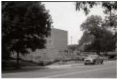
Demolition of 1110 and 116 Quincy Street (250-05-01-3542)
