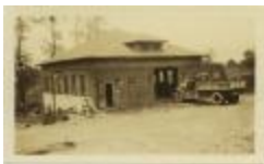
Farm Repair Shop (32-07-08-02-0167)
