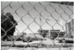
Construction on Wilson (250-09-01-8788)
