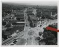
Proposed Site for Central Library Branch Location (29-01-13-01-0268)
