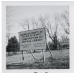
Arlington Central Library Construction (29-01-13-01-0058)
