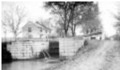
C&O Canal Lock and Lockhouse (123-02-03-0155)
