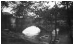
An Aqueduct of the C&O Canal (123-02-03-0098)
