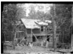
The Jewett Home Under Construction (123-02-06-0077)
