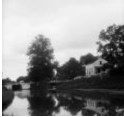
Lock and Lockhouse on C&O Canal (123-02-03-0109)
