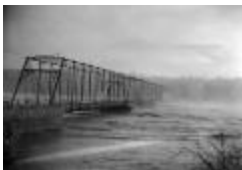
Chain Bridge Flood (123-02-02-0087)
