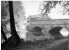
An Aqueduct of the C&O Canal (123-02-03-0096)
