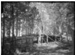
Frame of the Jewett Home Under Construction (123-02-06-0071)
