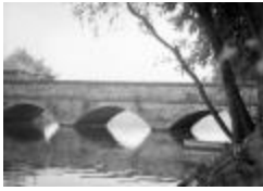
An Aqueduct of the C&O Canal (123-02-03-0102)
