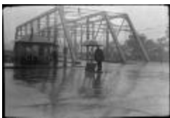
Aqueduct Bridge at 36th and M (123-02-02-0088)
