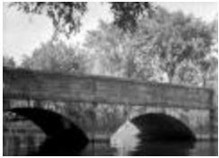
An Aqueduct of the C&O Canal (123-02-03-0093)
