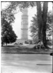
Washington Monument Under Construction (123-02-16-0048)
