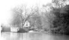
C&O Canal Lock and Lockhouse (123-02-03-0152)
