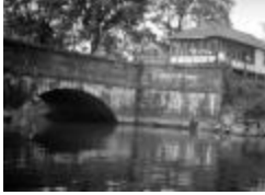
An Aqueduct of the C&O Canal (123-02-03-0101)
