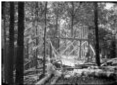
Frame of the Jewett Home Under Construction (123-02-06-0070)
