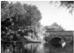
An Aqueduct of the C&O Canal (123-02-03-0097)
