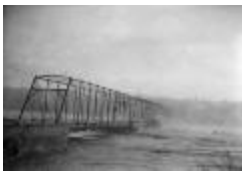
Chain Bridge Flood (123-02-02-0086)
