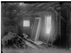
Interior of the Jewett Home Under Construction (123-02-06-0078)
