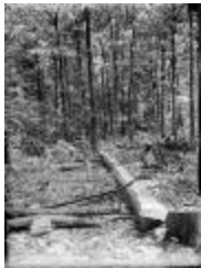
Cleared Area for the Jewett Home (123-02-06-0074)
