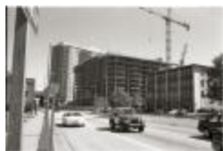
Construction on Fairfax Drive (250-09-01-8792)
