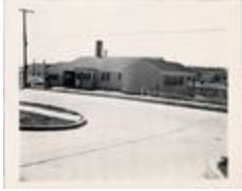
Dunbar Health Center, 3500 South Kemper Road, 1958 (21-5442)
