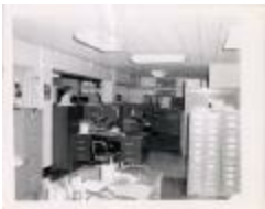
Courthouse Basement, South Wing, IBM section (100-03-01-0425)
