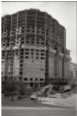
Construction of Arlington Courthouse Place (250-03-01-2884)
