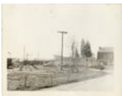
Trailer Camp Health Center, 1943 (21-5318)
