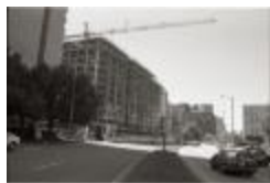
Construction on Fairfax Drive (250-09-01-8791)
