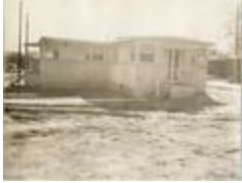
Trailer Camp Health Center (21-5208)
