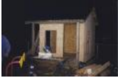
Construction at Night (332-05-08-0133)
