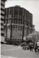
Construction of Arlington Courthouse Place (250-03-01-2883)
