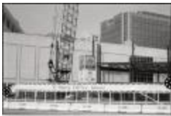
Hecht Company Office Tower Construction (250-05-01-3550)
