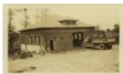
Farm Repair Shop (32-07-08-02-0167)
