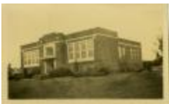
Henry Clay School Building (32-07-08-01-0139)
