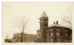
Arlington County Courthouse (100-03-01-0401)
