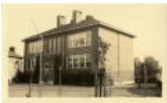
New Cherrydale School Building (32-07-08-01-0137)
