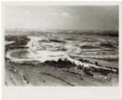
Construction of Washington National Airport (13-06-03-5084)
