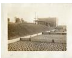
"Laboratory Disposal Plant" (21-01-01-13-5154)
