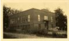
Kemper School Building (32-07-08-01-0146)
