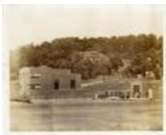
Water Pollution Control Plant (21-01-01-13-5153)
