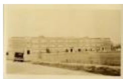
Washington-Lee School Building (32-07-08-01-0154)
