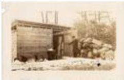
Inspection of Garbage (21-01-01-15-5168)
