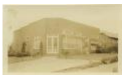
Virginia Highlands Health Center (32-07-08-02-0171)
