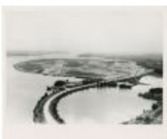
Construction of Washington National Airport from the North (13-06-03-5085)
