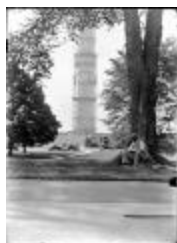
Washington Monument Under Construction (123-02-16-0048)
