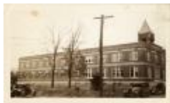
Arlington County Courthouse (100-03-01-0405)
