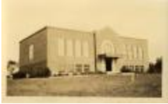
Barcroft School Building (32-07-08-01-0135)
