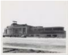
Construction of Terminal A (13-06-03-5099)
