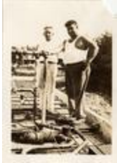
Inspection of Water Treatment Plant (21-01-01-15-5166)
