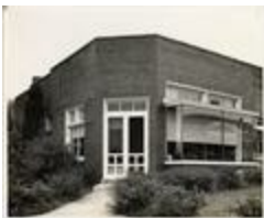
Jefferson District Health Center (21-01-01-08-5135)
