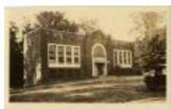
Woodmont School Building (32-07-08-01-0156)
