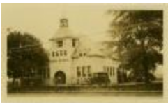
Hume School Building (32-07-08-01-0140)
