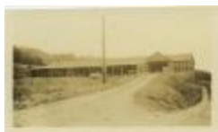
Farm Main Barn (32-07-08-02-0163)
