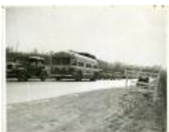
"Road Very Dangerous" (13-06-03-5110)
