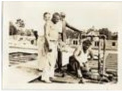
Inspection of Water Treatment Plant (21-01-01-15-5165)
