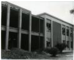
Building Addition Construction (214-01-01-9199)
