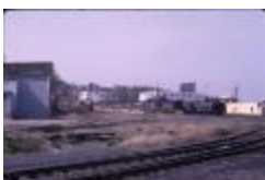
Rosslyn PA Freight Yard (210-0028)
