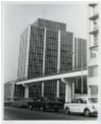
Rosslyn Pedestrian Bridge (214-03-01-9314)
