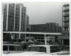
Rosslyn Pedestrian Bridge (214-03-01-9313)
