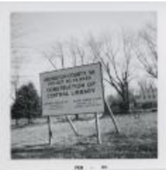
Arlington Central Library Construction (29-01-13-01-0058)
