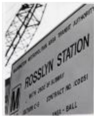
Rosslyn Metro Station Construction Sign (100-01-13-0266)
