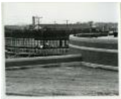
Working on the Water Pollution Control Center (214-01-03-9204)
