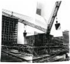
Copy of a Construction Site Photo (214-02-02-9242)
