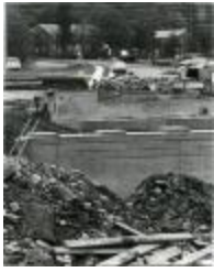
Construction Site with Neighborhood in Background (214-01-01-9200)
