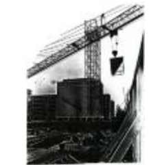
Copy of a Construction Site Photo (214-02-02-9240)
