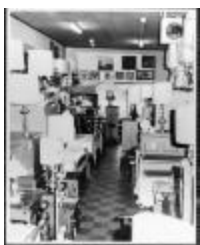
Columbia Furniture, Interior View (212-8729)
