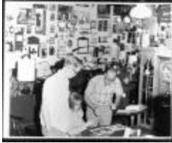
Columbia Furniture, Interior View (212-8731)
