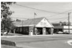
Arlington County Fire Station 6 Falls Church, 1996 (202-6145)
