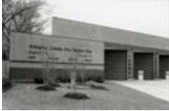
Arlington County Fire Station 1 Glebe Road, 1996 (202-6138)
