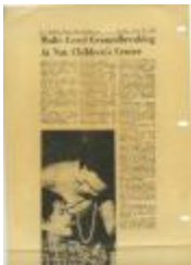
Northern Virginia Sun March 23, 1972 "Syphax Groundbreaking National Children's Center" (196-03-23-1972)
