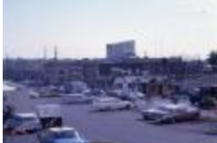
Shops at the Base of Key Bridge in Rosslyn (210-0019E)
