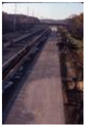
I-66 and Metro Construction (210-0048)
