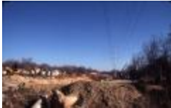
Construction of I-66 Near McKinley Road (210-0012)
