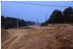
Construction of I-66 from the Patrick Henry Overpass (210-0014)
