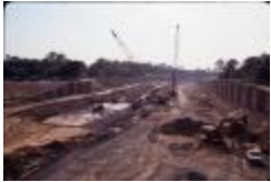
Construction of I-66 (210-0046)
