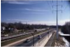
Completed I-66 Near Westover Baptist (210-0013)
