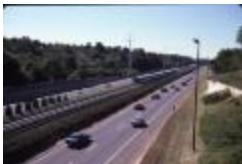
Completed I-66 from the Patrick Henry Overpass (210-0015)
