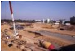
Construction of I-66 in Ballston (210-0001)
