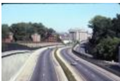
Completed Section of I-66 Going Through Rosslyn (210-0016)
