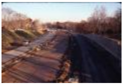
Construction of I-66 from the Patrick Henry Overpass (210-0047)
