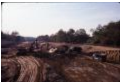
Construction of I-66 (210-0043)
