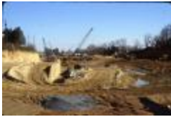
Construction of I-66 from the Harrison Street Bridge (210-0044)
