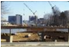
Construction of the George Mason Bridge (210-0042)
