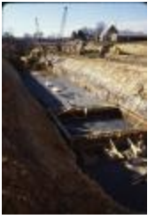
Pouring Concrete for I-66 (210-0045)
