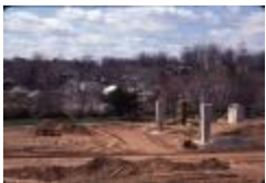
Construction of the Pedestrian Overpass at N. Potomac Street (210-0049)
