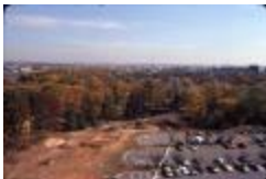
Construction Area of I-66 from Above (210-0009)
