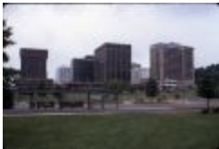
Rosslyn Circle Bus Terminal (210-0029)
