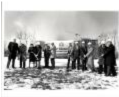
Groundbreaking C&P Telephone company building at Courthouse Plaza (333-07-03-0044)
