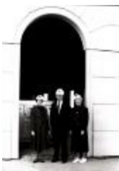
Bozman at Courthouse Plaza Construction (333-07-03-0040)
