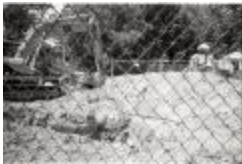
Fixing Water Main at Woodmont (250-05-01-3540)
