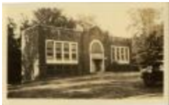
Woodmont School Building (32-07-08-01-0156)
