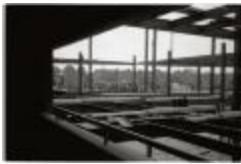
Hecht Company Office Tower Construction (250-05-01-3547)
