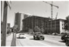
Construction on Fairfax Drive (250-09-01-8792)
