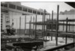
Hecht Company Office Tower Construction (250-05-01-3548)
