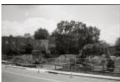
Demolition of 1110 and 116 Quincy Street (250-05-01-3543)
