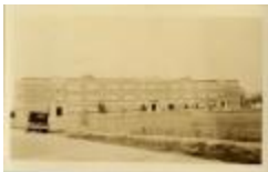
Washington-Lee School Building (32-07-08-01-0154)
