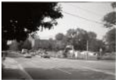
Construction on Quincy Street (250-05-01-3554)
