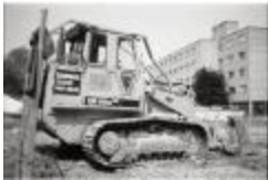
Dominion Front Loader on Site (250-05-01-3558)
