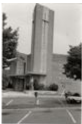
St. Charles Borromeo Catholic Church, 1996 (202-6101)
