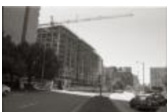
Construction on Fairfax Drive (250-09-01-8791)
