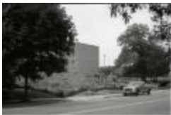
Demolition of 1110 and 116 Quincy Street (250-05-01-3542)
