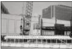
Hecht Company Office Tower Construction (250-05-01-3550)
