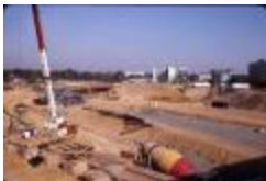
Construction of I-66 in Ballston (210-0001)
