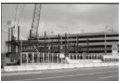
Hecht Company Office Tower Construction (250-05-01-3551)
