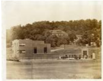
Water Pollution Control Plant (21-01-01-13-5153)
