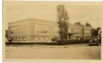
Nellie Custis School Building (32-07-08-01- 0148)
