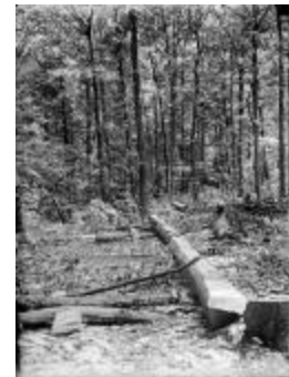
Cleared Area for the Jewett Home (123-02-06-0074)
