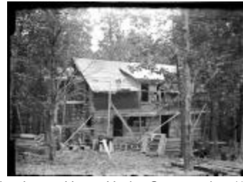
The Jewett Home Under Construction (123-02-06-0077)
