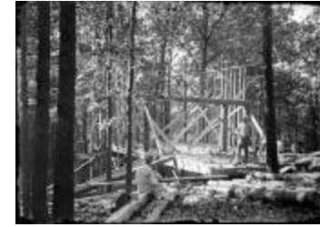
Frame of the Jewett Home Under Construction (123-02-06-0070)
