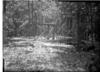
Frame of the Jewett Home Under Construction (123-02-06-0068)
