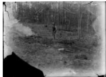
Construction Worker on Jewett Home Lot (123-02-06-0072)
