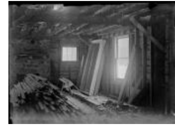
Interior of the Jewett Home Under Construction (123-02-06-0078)
