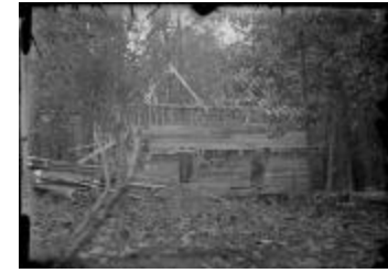
The Jewett Home Under Construction (123-02-06-0066)
