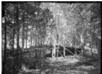
Frame of the Jewett Home Under Construction (123-02-06-0071)
