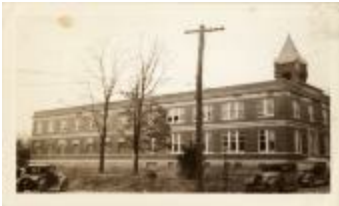
Arlington County Courthouse (100-03-01-0405)
