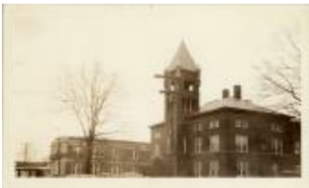
Arlington County Courthouse (100-03-01-0401)
