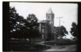
Arlington County Courthouse (100-03-01-0403)
