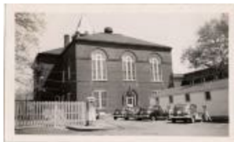
Arlington County Courthouse (100-03-01-0416)
