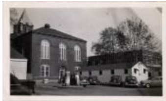
Arlington County Courthouse (100-03-01-0408)
