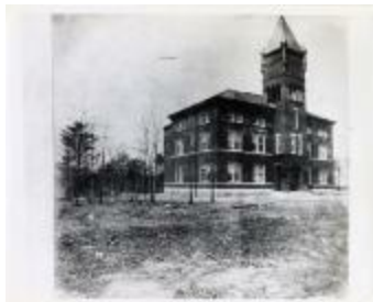
Arlington County Courthouse (100-03-01-0402)
