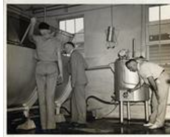
Inspection of Pasteurizing Plant (21-01-01-13-5157)
