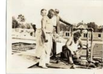
Inspection of Water Treatment Plant (21-01-01-15-5165)
