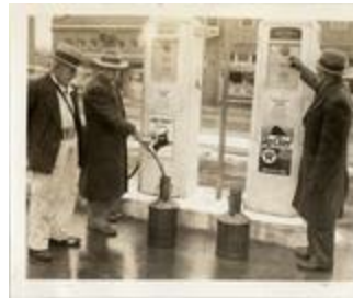
Inspection of Gasoline Pump (21-5253)
