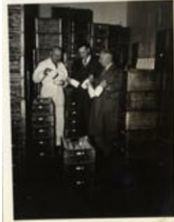
Inspection of Milk Storage Facility, 1943 (21-5304)
