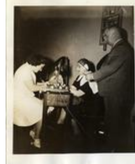
Inspection of Beauty Parlor, 1943 (21-5319)
