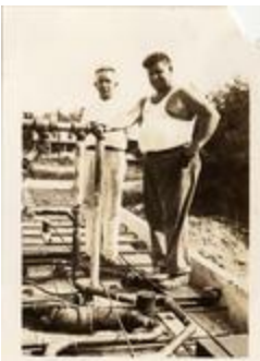
Inspection of Water Treatment Plant (21-01-01-15-5166)
