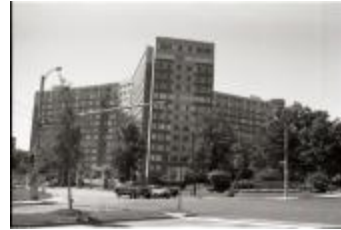
Riverhouse Apartment Building (250-09-01-8785)
