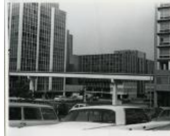
Rosslyn Pedestrian Bridge (214-03-01-9313)
