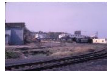
Rosslyn PA Freight Yard (210-0028)
