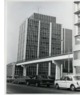
Rosslyn Pedestrian Bridge (214-03-01-9314)
