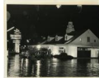
Flooding at Hot Shoppes (214-04-04-9367)
