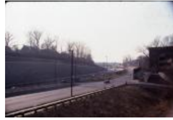
Finished I-66 West Out of Rosslyn (210-0037)
