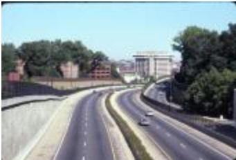
Completed Section of I-66 Going Through Rosslyn (210-0016)
