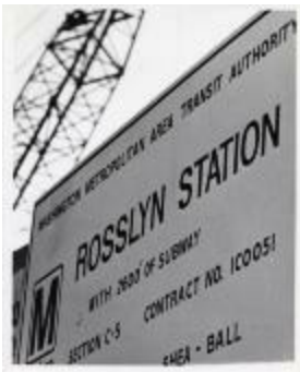
Rosslyn Metro Station Construction Sign (100-01-13-0266)
