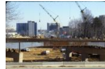
Construction of the George Mason Bridge (210-0042)
