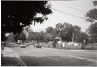
Construction on Quincy Street (250-05-01-3554)
