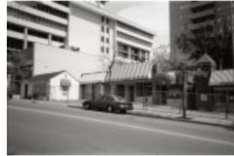
Closed Strip Mall on Courthouse Road (250-03-01-2881)
