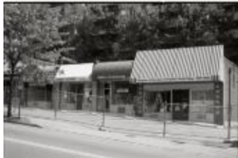
Closed Strip Mall on Courthouse Road (250-03-01-2879)
