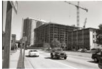
Construction on Fairfax Drive (250-09-01-8792)
