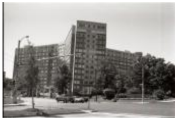
Riverhouse Apartment Building (250-09-01-8785)
