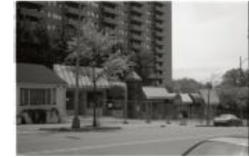
Closed Strip Mall on Courthouse Road (250-03-01-2882)
