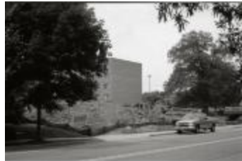
Demolition of 1110 and 116 Quincy Street (250-05-01-3542)
