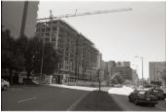
Construction on Fairfax Drive (250-09-01-8791)
