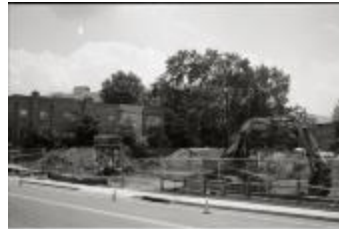
Demolition of 1110 and 116 Quincy Street (250-05-01-3543)
