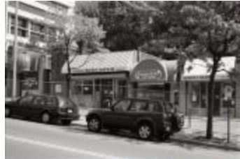
Closed Strip Mall on Courthouse Road (250-03-01-2880)
