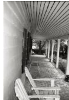
Basil Hall House Front Porch (250-08-01-8766)
