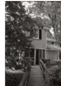
Kitchen Entrance to Basil Hall House (250-08-01-8767)
