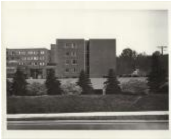
Hospital From Street, Garage (32-04-11-12-0120)
