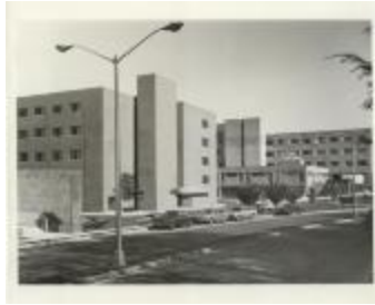
Hospital From Street, Two Light Poles (32-04-11-12-0121)
