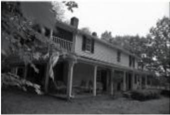
Basil Hall House Front Porch (250-08-01-8747)
