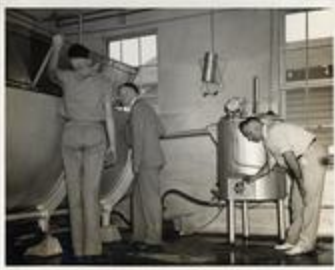
Inspection of Pasteurizing Plant (21-01-01-13-5157)
